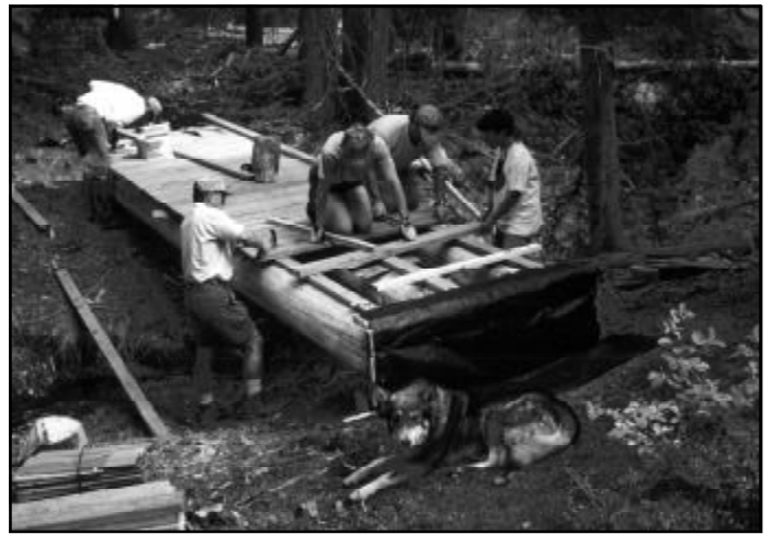
Volunteers building the first bridge across Sawmill Creek.
